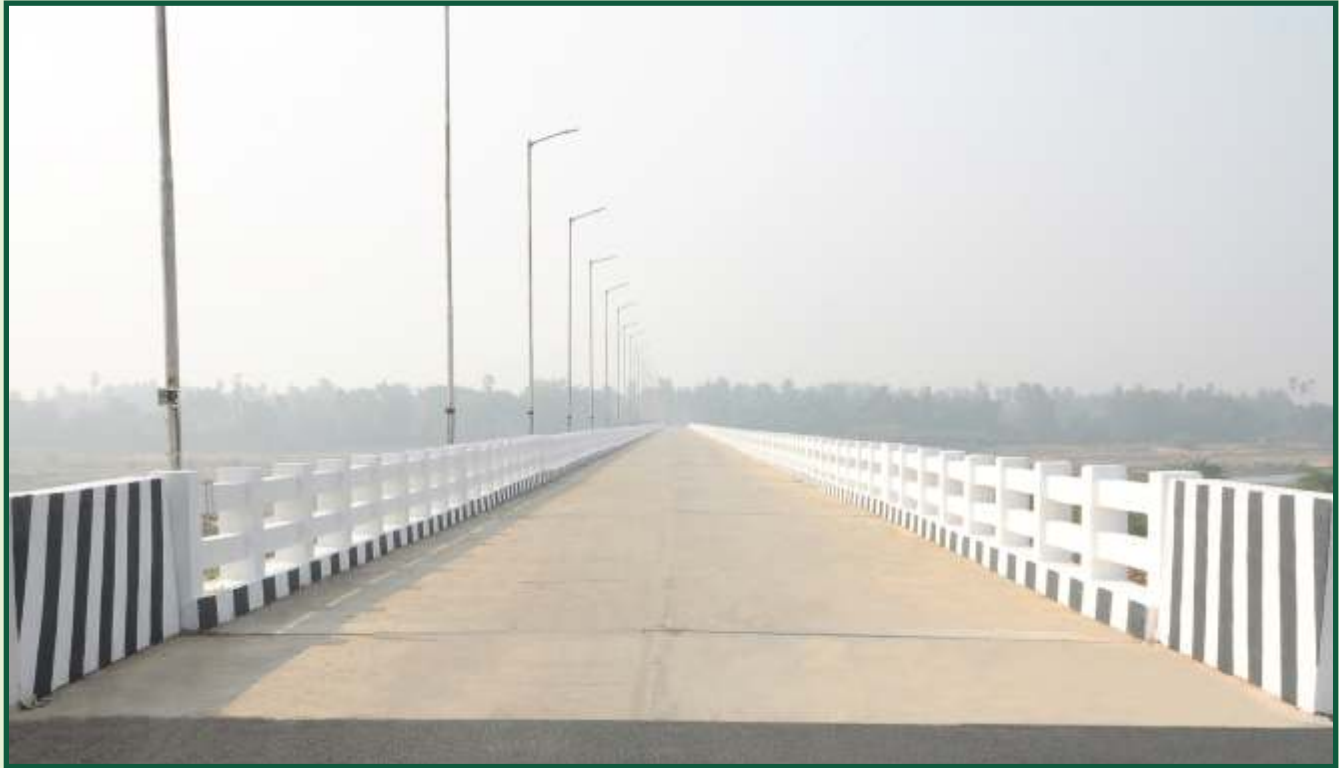
Construction of New Bridge
