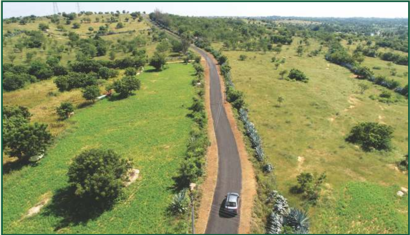
Formation of Black Topped Road
